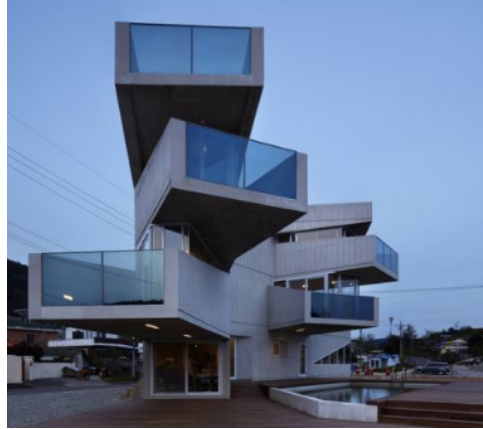
Figure 10. Projecting Roofs or Floors
